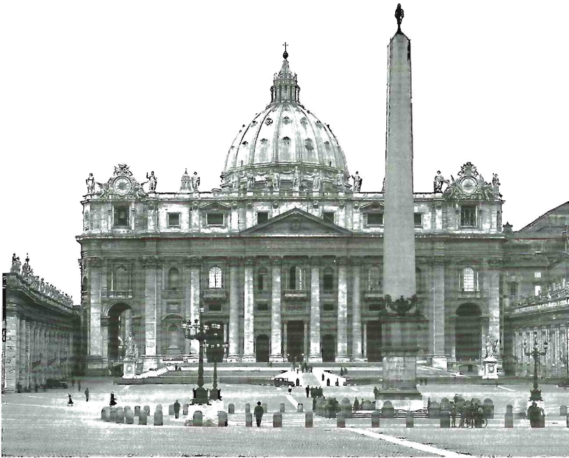
Fig. 5. Facade of Saint Peter's Basilica. Vatican City.
