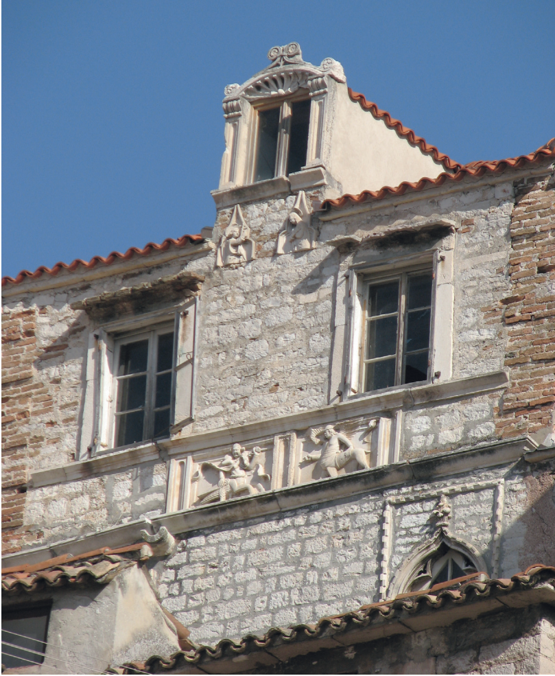
FIG. 9 Window Detail, c. later 15th century, Sebenico (PHOTO BY THE AUTHOR).
