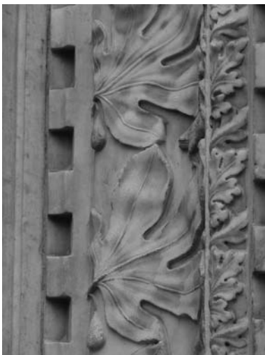
Fig. 14. Detail of marble doorframe, South transept portal, Duomo, Florence. (Photo by: Alina Payne.)
